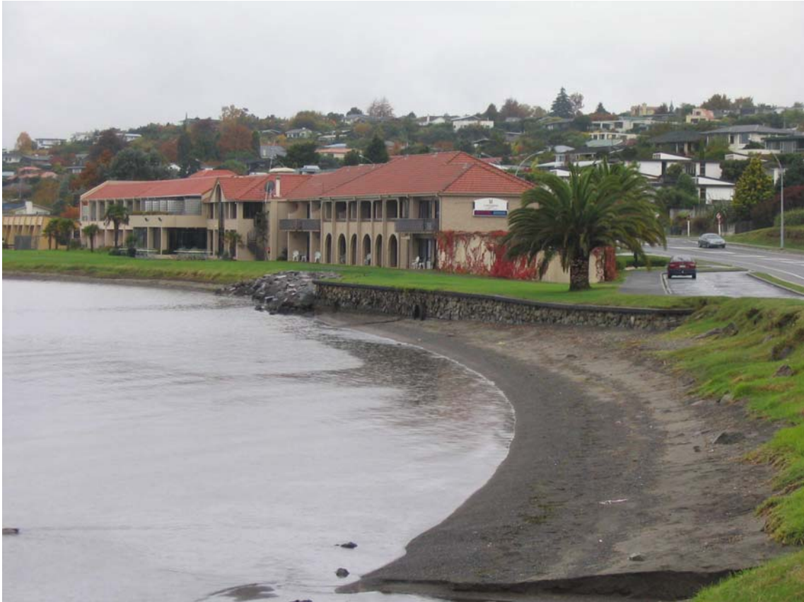
Photo 11. Taupo Township mix of structures, May 2005
